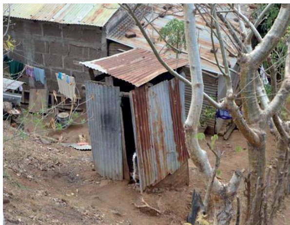
FIGURE 4.1: LATRINE ON THE OUTSKIRTS OF SANTA CRUZ
