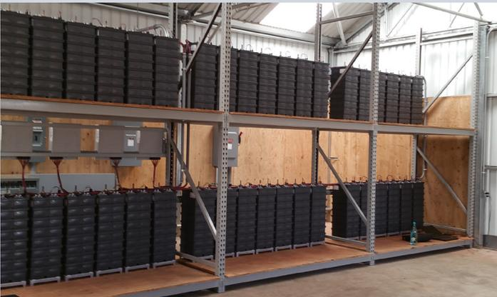
*Forty Aquion battery stacks are used to power a 25-kilowatt installation at Mari's Garden, a nursery in Millani, Hawaii. The business's heavy power demand – combined with high Hawaiian electricity costs – made combining a solar PV array with Aquion batteries a smart financial decision. (Photo courtesy of Aquion)*
